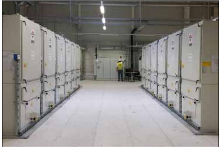
Central separation system with twelve AERO® modules, size 3
